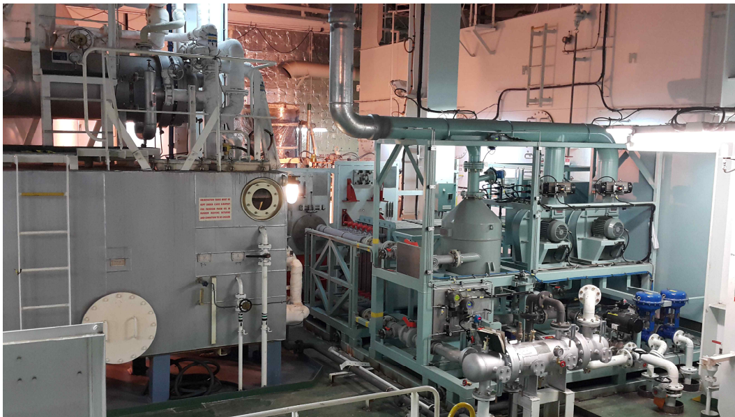
[Fig. 44] Example for typical field installation of BWMS using Electrolysis technology (Side-stream type)
