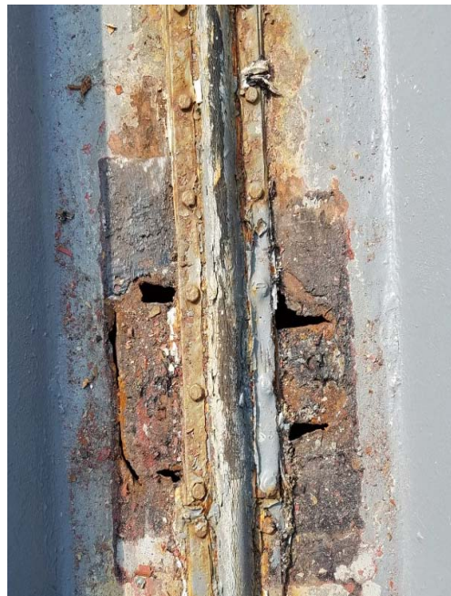
[ Holed and Corroded ]
