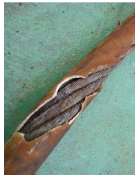
Figure 2. Corrosion beneath plastic sheathing.
