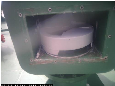
Damaged plastic disk
